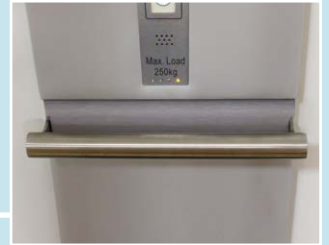
straight stainless steel hand rail
